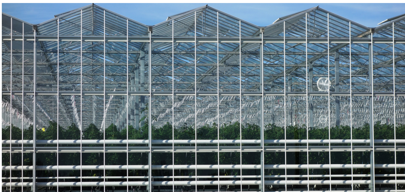
Figure 1 - A view of the exterior of a Dutch Venlo greenhouse used to grow vine crops hydroponically. The greenhouses will be visible from Kostner.
