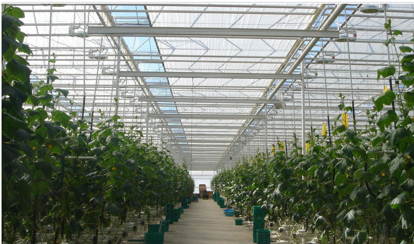
Figure 2 - An interior view of a Dutch Venlo greenhouse, with vine crops growing vertically, with its horizontal solar screens deployed.
